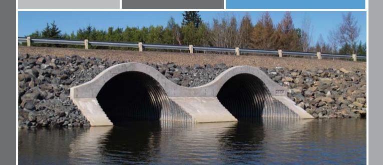
**High Profile** arches are engineered to maintain a natural waterway and allow for an abrasive bedload. Additionally, these arches are ideal for projects that include large end areas or large spans. The high profile arch is also used for highway grade separations.
