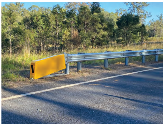
The MAX-Tension Energy Absorbing Coupler (gold) is fitted with a patent pending galvanized Sabertooth (red). When the system is impacted head-on, the Sabertooth is engineered to cut the downstream guardrail to aid in the deceleration of an errant vehicle.
